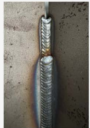
WELDING IN CONSTRAINED POSITIONS
